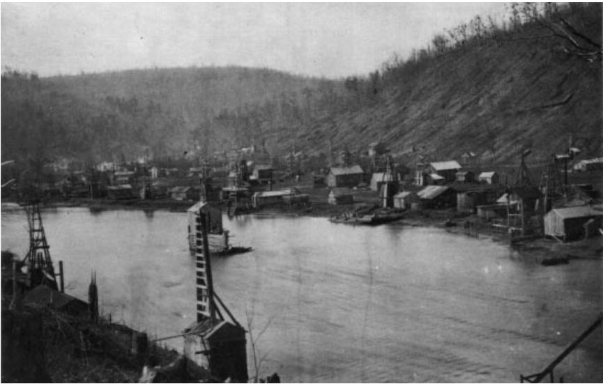
Figure 2. A well believed to be in the locality of the Hamilton McClintock seep in the middle of Oil Creek. The V has snagged some driftwood. Photograph courtesy of the Drake Well Museum.
