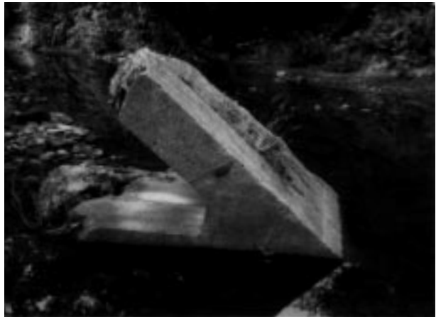
Figure 3. A concrete V pointing upstream at Pioneer. This barricade has been shifted by floods and ice-outs. A well was drilled behind the V and originally was protected by it. The island was created by the reduction of flow velocity behind the V.
