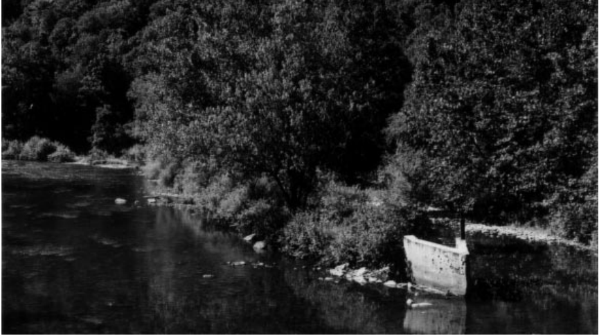
Figure 3. A concrete V pointing upstream at Pioneer. This barricade has been shifted by floods and ice-outs. A well was drilled behind the V and originally was protected by it. The island was created by the reduction of flow velocity behind the V.
