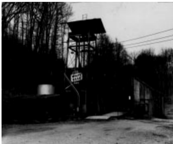
Figure 3. The Venango Development Corporation oil mine near Franklin as it looked in 1960. The tower supported the pipelines and elevator shaft. Photograph by William S. Lytle.
