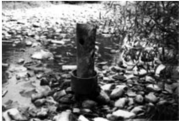
Figure 5. A pier jutting into Cherrytree Run, a tributary of Oil Creek. Note the Oklahoma-type pumping jack. This pier well can produce from the Venango Second sand. Photograph by Ellsworth “Pete” Sparks.
