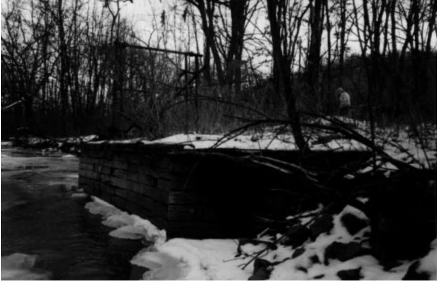
Figure 5. A pier jutting into Cherrytree Run, a tributary of Oil Creek. Note the Oklahoma-type pumping jack. This pier well can produce from the Venango Second sand. Photograph by Ellsworth “Pete” Sparks.
